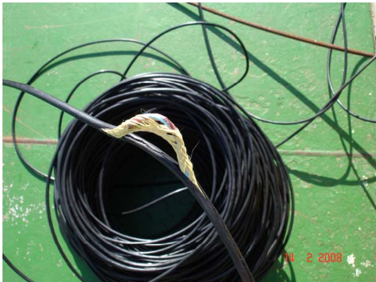
Fig 1. SPMR cable cut during recovery.
